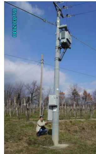
Fig. 4.4: Pole-mounted transformer substation with an unprotected transformer.
