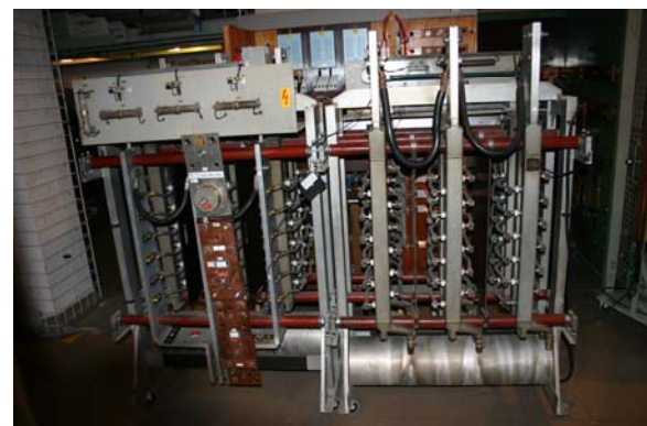
Fig 4: Temporary rectifier from TALUM
