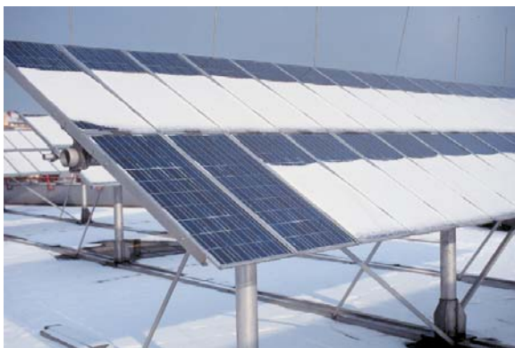
Fig. 3.2: Solar generator partially covered by snow
