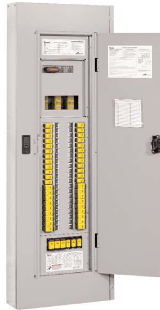
Fig. 13: This figure shows a 200 ampere, 600 volt panelboard with a 200 ampere main fused switch with 200 ampere Class J time-delay fuses. Spare fuses are located in the horizontal row across the bottom of the panel. Panel can have either a 50kA or 200kA short-circuit current rating.
