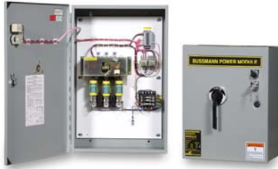
Fig. 4: This figure shows a fusible disconnect switch with shunt-trip capability so that all power to the elevator can be removed before the application of water in the elevator shaft.
