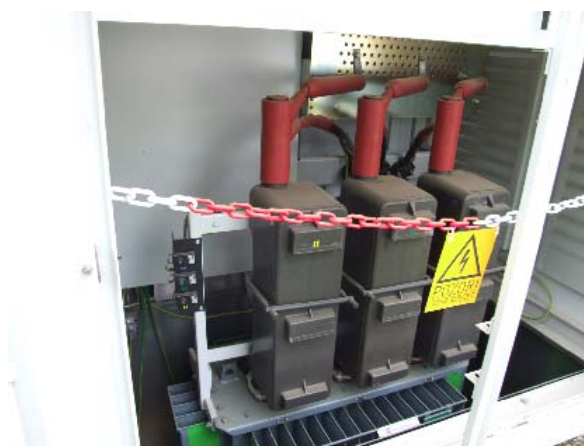
Figure 14: An example of application of fuse holder type VOH1, which insulates the HV part in a transformer substation
