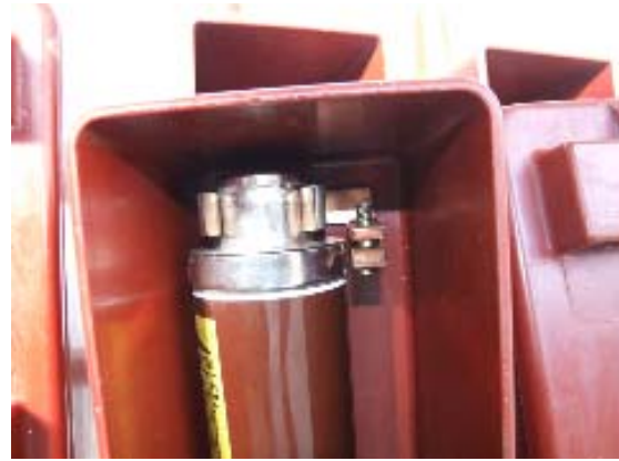
Figure 6: Detail of upper contacts
