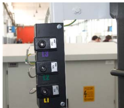
Figure 2: Voltage indication on VOH 01 carried out with IN5
