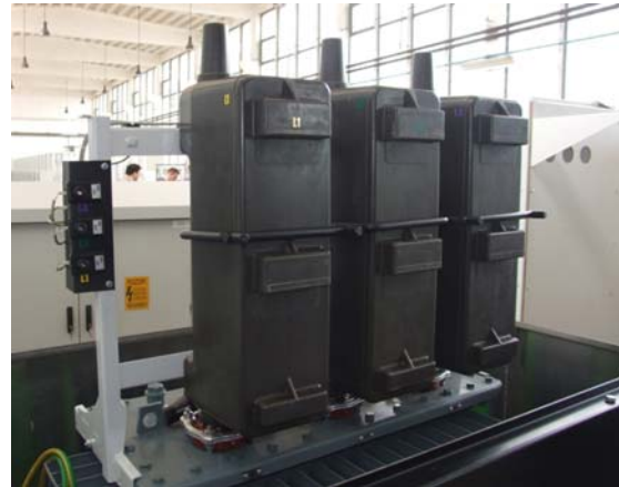
Figure 1: Insulated HV fuse holder VOH 01 (design by TSN) mounted on a transformer's cover (50 kVA).
